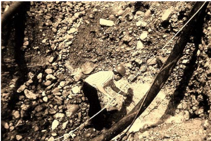
Figure 7 Clay layer within gravel
